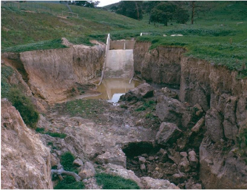
SCA gully erosion control structure
