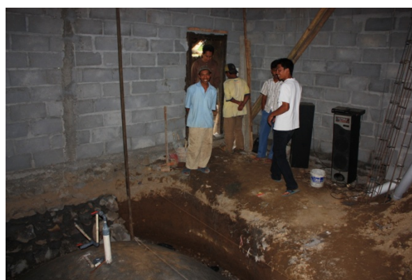
Biogas installation under construction. Photo: SILC Nov. 2013
