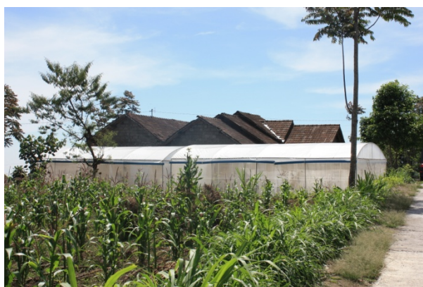
New Hot house constructed beside the Landcare Centre. Photo: SILC Nov. 2013
