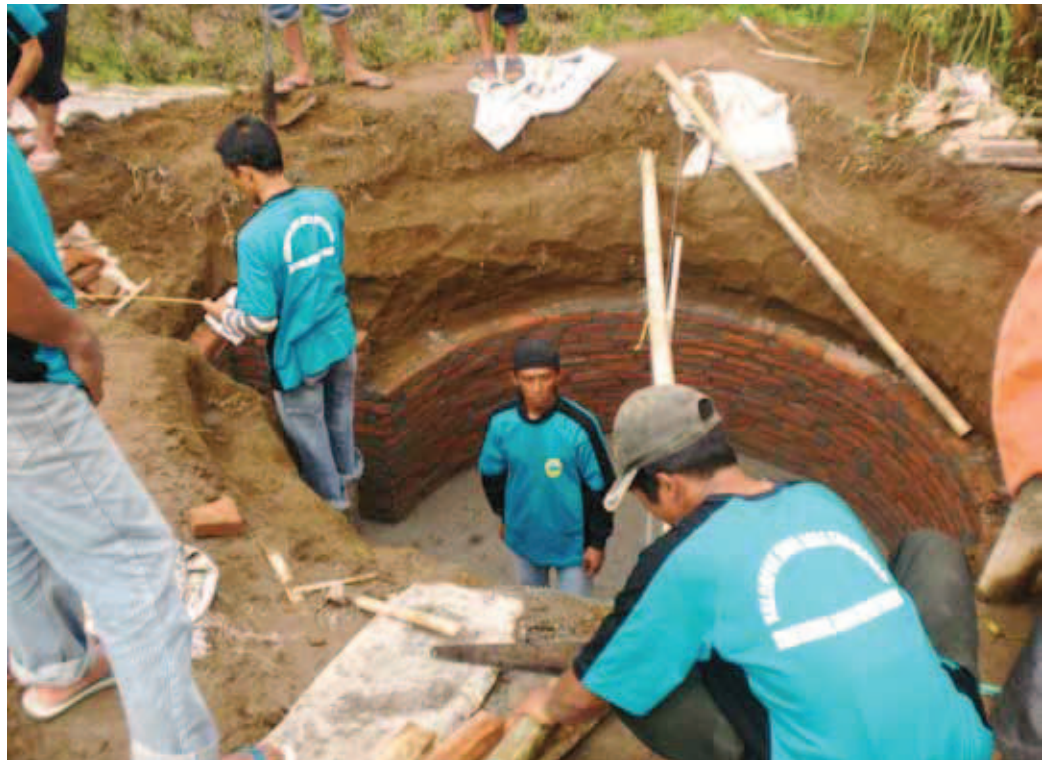
Volunteers from Merapi Landcare construct a biogas digester.
